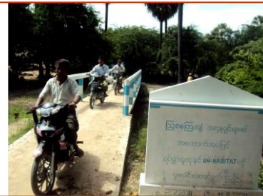
Small Bridge Construction
