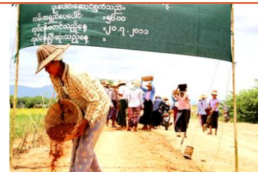
Feeder Road Upgrading
